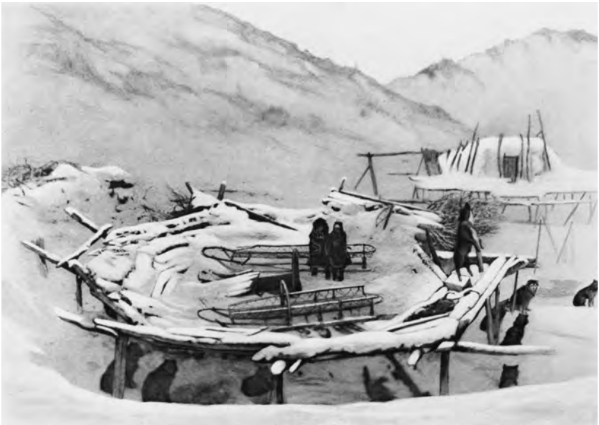
Fig. 2. View of Storm-Roof.
