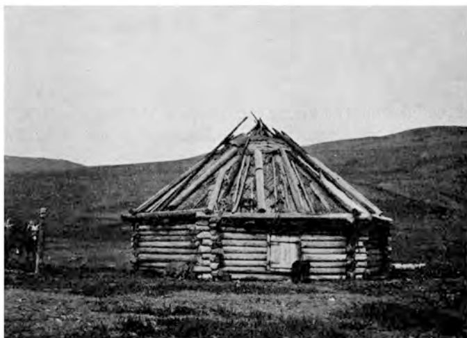
Fig. 25. Polygonal Sloping Roofed Blockhouse at Verkhne Kolymsk.
